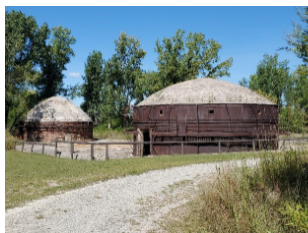
Historic Kilns used to fire bricks and drain tiles at the old Rockford Brick and Tile Company at the present-day Floyd County Fossil and Prairie Park. (Lowell Hill)
