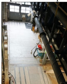
Figure 7a: The bottom floor of SAFL that has been known to flood during high water. (John Foley)
