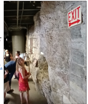
Figure 7b: Dolomitic limestone bedrock forms the lower walls of SAFL. This stone was mined on site to build the laboratory. (John Foley)
