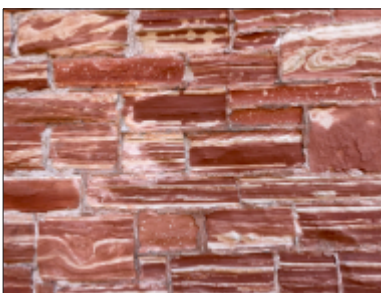
Neoproterozoic Jacobsville Sandstone used in the smelter was locally quarried. The red oxidation developed after deposition in relation to fluids. The white spots and layers are high in organic material that prevented oxidation. The cross-bedding and channels indicate a fluvial origin. (K. Clover)
