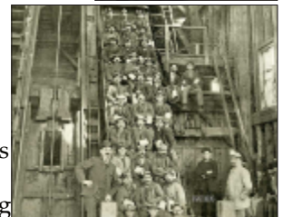
Miners in a man car at the Quincy No. 2 Shaft/Rock House, ready to go underground. In 1945, the No 2 shaft had reached 9260 feet, the longest mine shaft in the world at the time. Miners used candles or oil lamps for light underground during this period; later, they used carbide or electric lamps. (Michigan Technological University archives, Copper Country Historical Collections).
