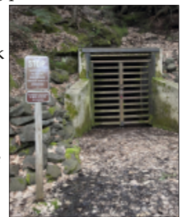
The Adventure Mine adit has a grated door that allow bats to come and go. Yes, we saw bats underground. (K. Clover)
