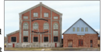
The 5-story Quincy Hoist building housed the cable hoist drum of the 1920 Norberg Steam Hoist. (K. Clover)
