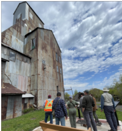
The Champion No. 4 Shaft/Rock House, built in 1902, is the oldest remaining shaft/rock house in the Copper Country. It operated from 1902 to 1928 and again from 1945 until 1967, when the mine ceased operations and the structure was abandoned intact with much of the equipment in position. The shaft was capped in 1995, and a bat door allows access. (K. Clover)
