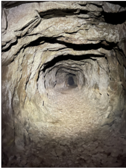
Looking down a mine adit with a ceiling 3' to 6' high. (K. Clover)
