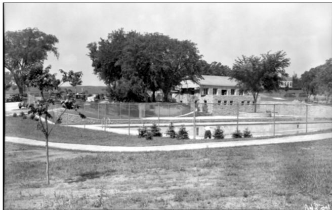
Figure 7. The concrete-lined rectangular Highland Pool, built by the WPA and opened in 1936, replacing the much larger "swimming hole." Courtesy of MHS.
