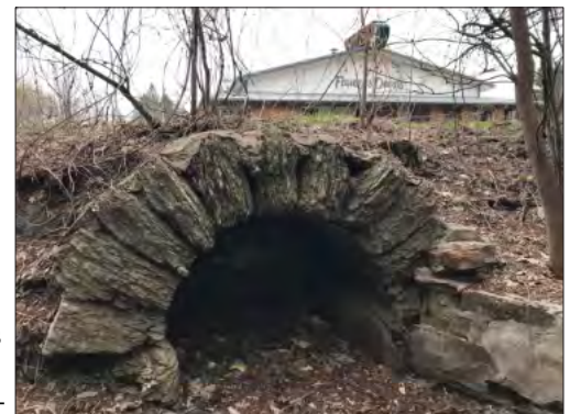
Figure 13a. Stone culvert under Fort Road, photo by author, 2023.
