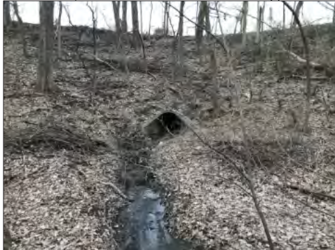
Figure 11b. The Highland Creek outfall reunites drainage from the upper, middle, and lower portions of the original watershed, before flowing into the Mississippi River. Photos by author, 2023.
