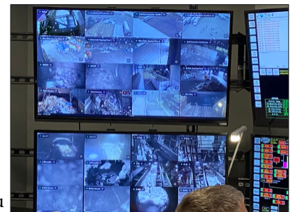
The control room operator monitors the video feeds from the cameras in and around machinery in the facility
