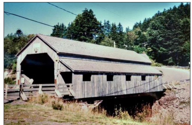
Covered bridge in St. Martins
