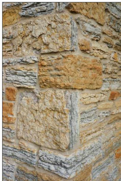
Stone blocks on the church were laid in various orientations. The stones vary in size.
