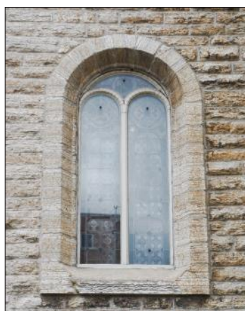
Window details of Assumption Church. Note the dressed stones framing the window.
