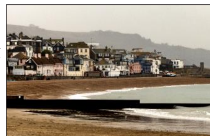
Lyme Regis from near The Cobb. The groyne in foreground prevents the beach beyond it from drifting eastward.
