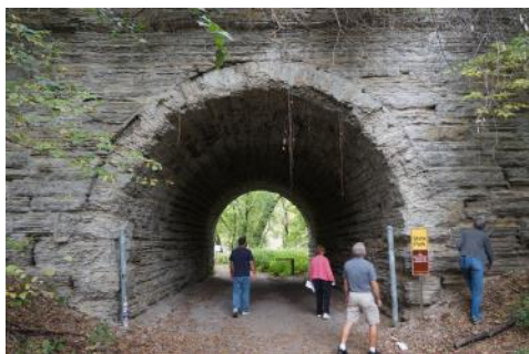
The rails over this 1864 bridge carried trains across the Minnesota River.
