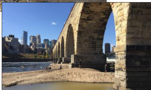
The darker lower portion of the piers of the Stone Arch Bridge; usually under water.
