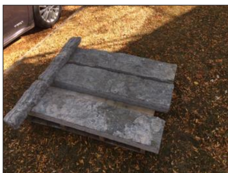
Replacement lintels for the Martin Weber house.
