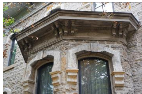
Stone around the windows on the Ramsey House was dressed and looks formal.
