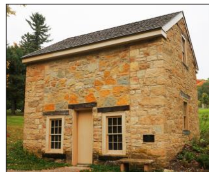
The icehouse next to the Sibley House shows multiple renovations.
