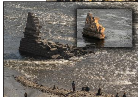
Remnants of a long-gone support, usually below the water line; inset shows same support at normal river level.
