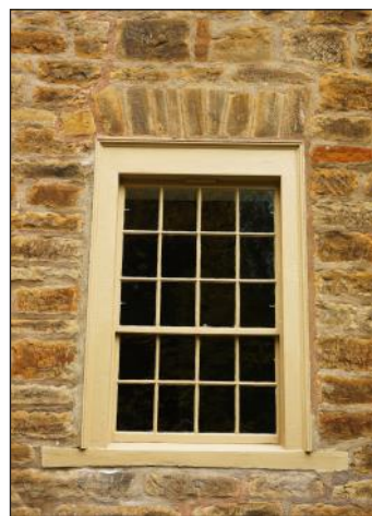
Stonemasons framed the top of the windows on the Faribault House with vertical stone blocks.
