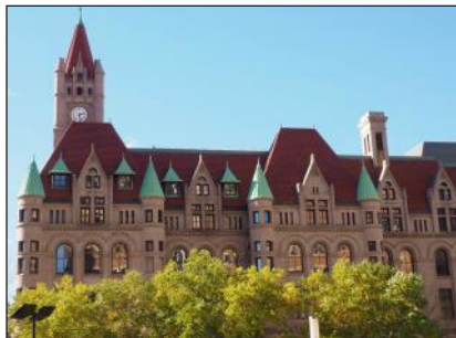
Landmark Center, completed in 1902, is built from Sauk Rapids pink granite. This building originally served as the Federal Court House and the Post Office, Customs and other Federal Agencies were housed here. This beautiful building survived demolition in the 1970s, and today is owned by Ramsey County and serves as a cultural center for music, dance, theater plus a couple of museums. Its exterior includes conical towers, turrets and gables. The interior features beautiful woodwork and stonework plus a five-story courtyard with a glass skylight.
