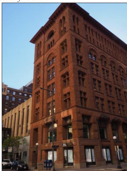
The eight-story St. Paul Building (Germania Bank) on the corner of 5th and Wabasha dates to 1890 and features deep red-brown Lake Superior sandstone with carved columns and pattern work. This stone is Jacobsville Sandstone from Michigan's Upper Peninsula.
