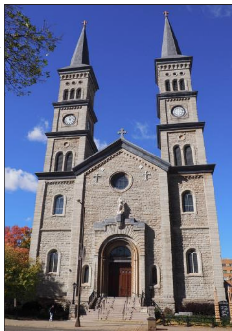
The Assumption Church on 7th Street dates to 1871. The limestone for this building was likely quarried on site and the stone is more precisely cut into blocks. Buildings of this style resembled others from that era.
