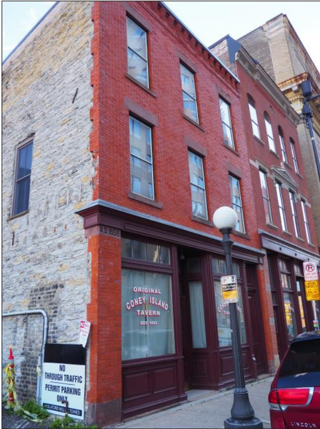
The Original Coney Island on St. Peter Street is two, side-by-side buildings that date to 1858 and 1888. The fronts on both are now faced with brick, but the sidewall shows the original limestone. This building illustrates and preserves the scale of buildings from this era.
