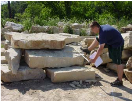
Conrad Zbikowski measures the chosen stone for installation at Beaver Creek Valley State Park
