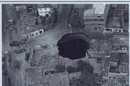
GUATEMALA CITY, Guatemala - A 330-foot-deep sinkhole killed at least two teenagers as it swallowed about a dozen homes in September and forced the evacuation of nearly 1,000 people in a crowded Guatemala City neighborhood. Officials blamed the sinkhole on recent rains and an underground sewage flow from a ruptured main. http://www.ordena.com/digg/sinkhole.html (suggested by Roger Knutson)
