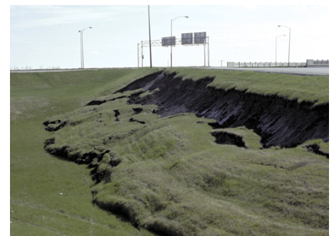
A land slump near Crookston (MGS Photo)
