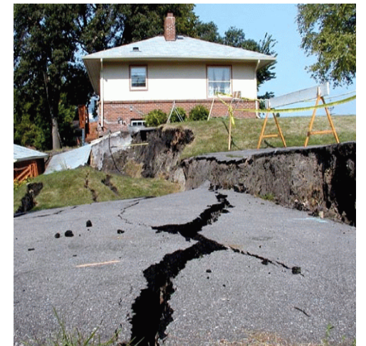
Riverbank failure sunk land by 3 feet in a Crookston neighborhood. Photo courtesy Crookston Daily Times.
